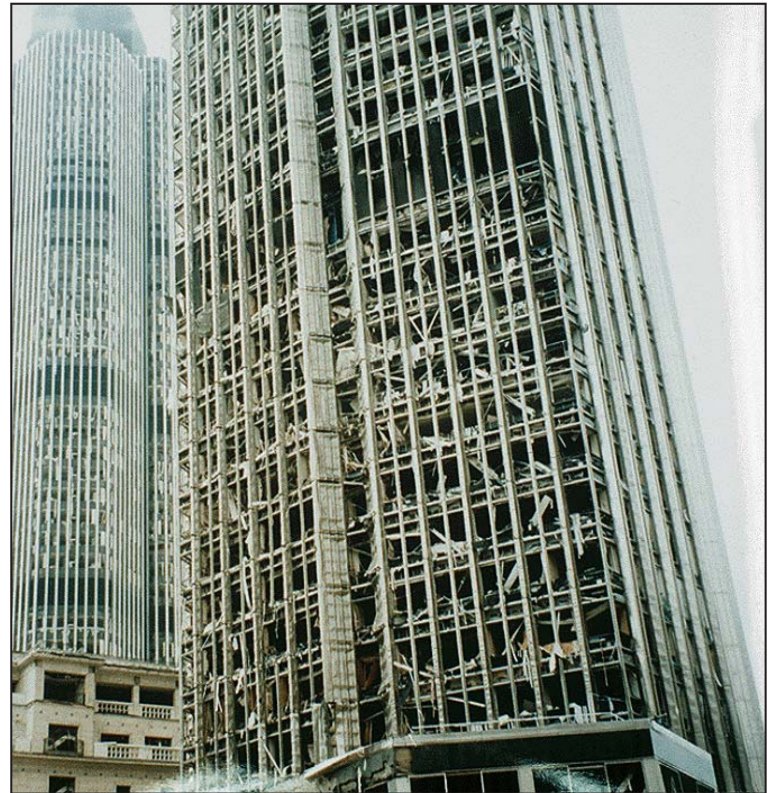
Thousands of windows were shattered by the Bishopsgate bomb, planted in London by the IRA in 1993.
